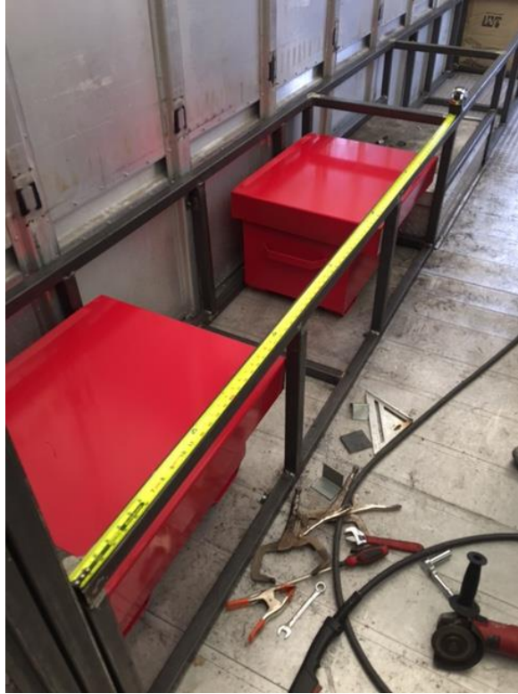
Figure 6 - Metal framing in the SWAT truck
