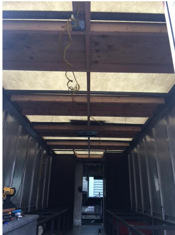
Figure 7 - Wiring and ceiling in the SWAT truck
