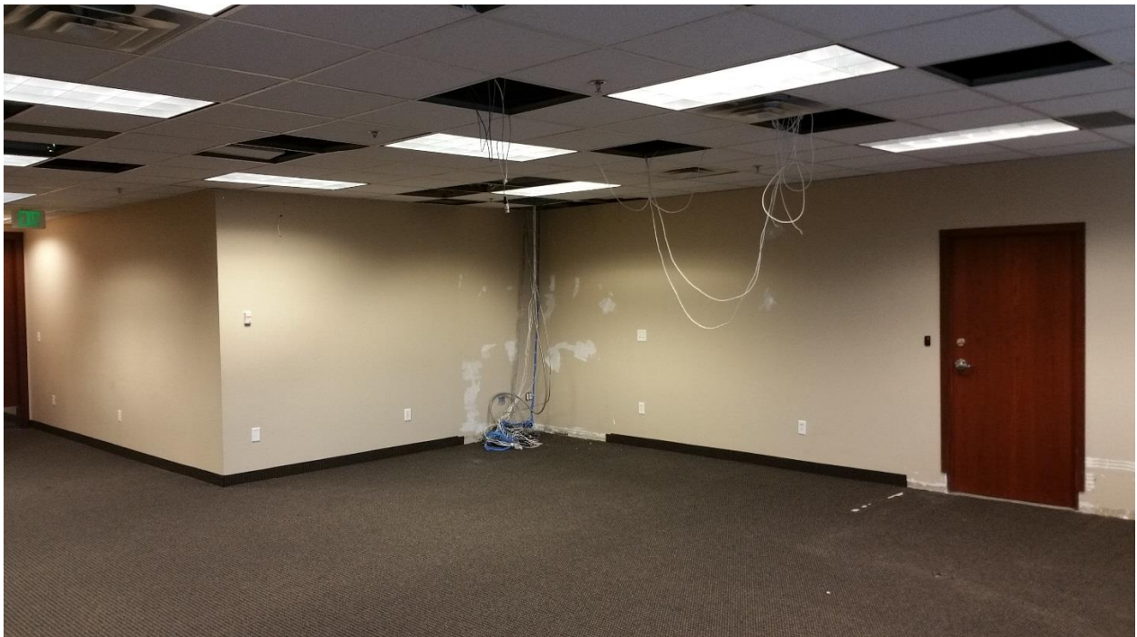
Figure 8 - Wiring needing to be removed from old council chambers
